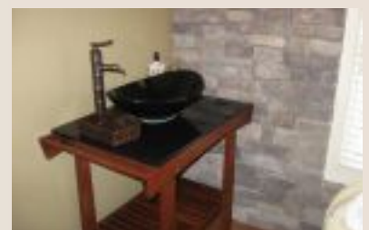
Installing the new wash basin for the massage area and adding the flooring and furnishings rounded out the project.
