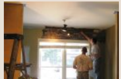
After the paint went up, it was time to install the stone finish on the accent wall.
