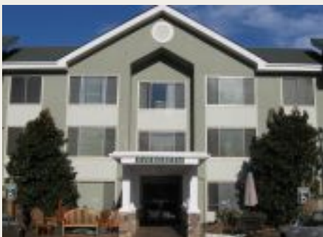
The installed windows and fresh paint are the perfect compliment to our mountaintop paradise.
