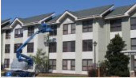
Our latest phase of renovation began with painting the building exteriors.
